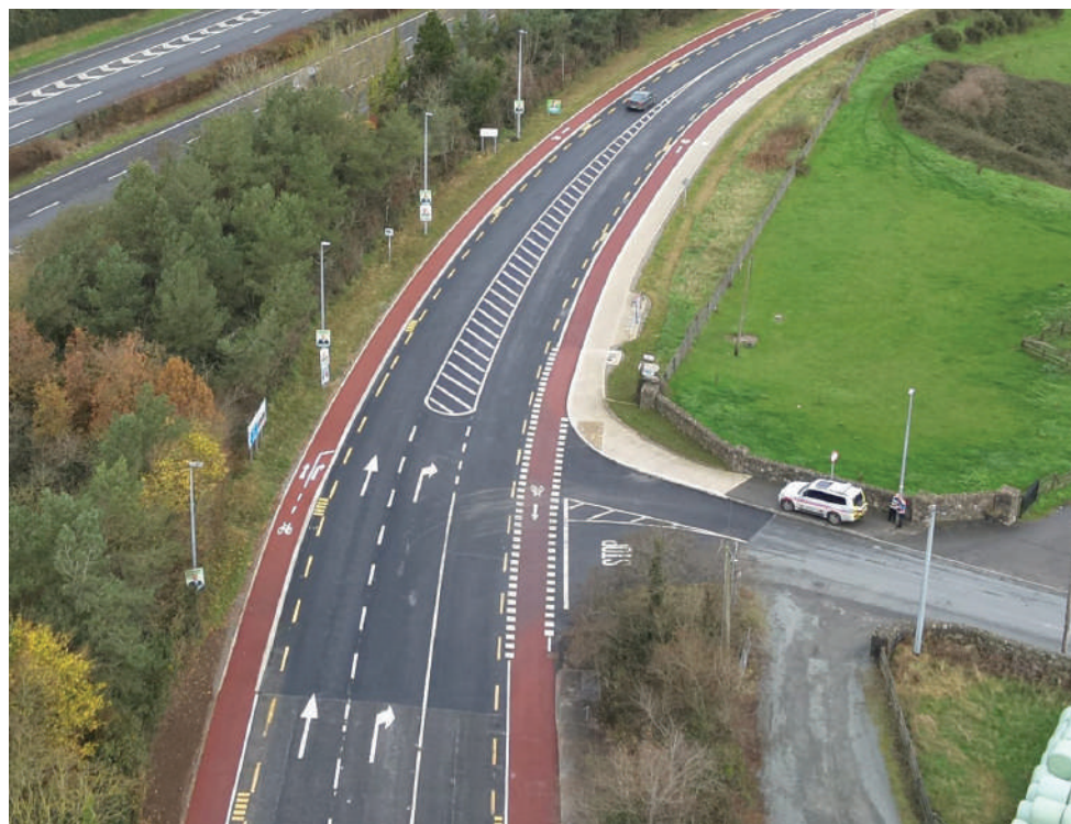
Recently finished Scheme at Arklow Road South R772.
