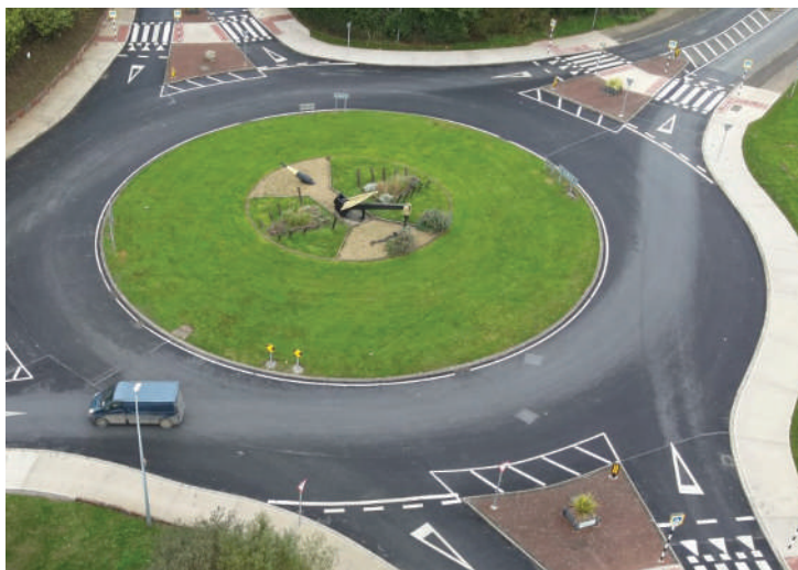
Roundabout at the recently finished scheme at Arklow Road South R772.
