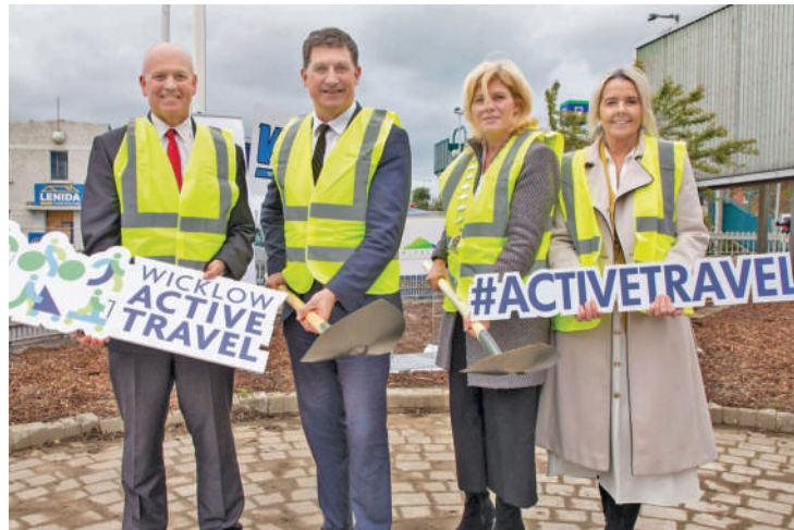
Pictured at the sod turning to mark the commencement of works for a transformative new Transport Hub in Bray on Thursday 18th April were (l-r) Michael Nicholson (Deputy Chief Executive Wicklow County Council), Minister of Transport Eamon Ryan TD, Cllr. Melanie Corrigan (Cathaoirleach of Bray Municipal District) and Lorraine Gallagher (District Manager of Bray Municipal District). Photo Mick Kelly
