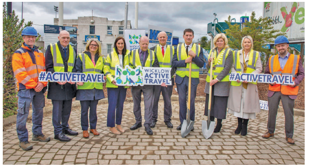
Pictured at the sod turning to mark the commencement of works for a transformative new Transport Hub in Bray on Thursday 18th April were (l-r) Joe Murphy (Project Manager, David Walsh Civil Engineering), Frank Masterson (Manager CIÉ Group Property), Finola O'Driscoll (Senior Programme Manager, NTA), Ursula O'Higgins (Technical Director, AtkinsRealis), Joe Lane, (Director of Services Infrastructure and Capital Projects Wicklow County Council), Michael Nicholson (Deputy Chief Executive Wicklow County Council), Minister of Transport Eamon Ryan TD, Cllr. Melanie Corrigan (Cathaoirleach of Bray Municipal District), Lorraine Gallagher (District Manager of Bray Municipal District) and Jamie Cassells (Contracts Manager, David Walsh Civil Engineering). Photo: Mick Kelly
