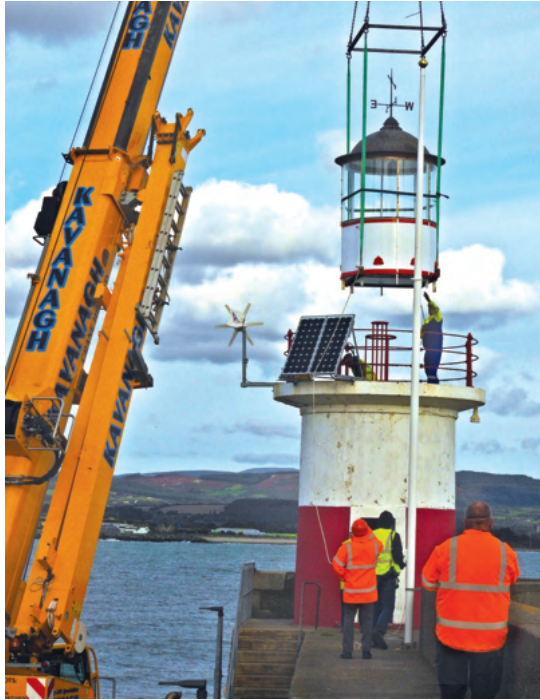
The roof being restored on the Wicklow East Pier lighthouse
