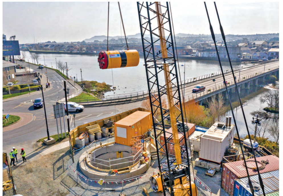
The tunnel boring machine being launched into the underground shaft in Arklow
