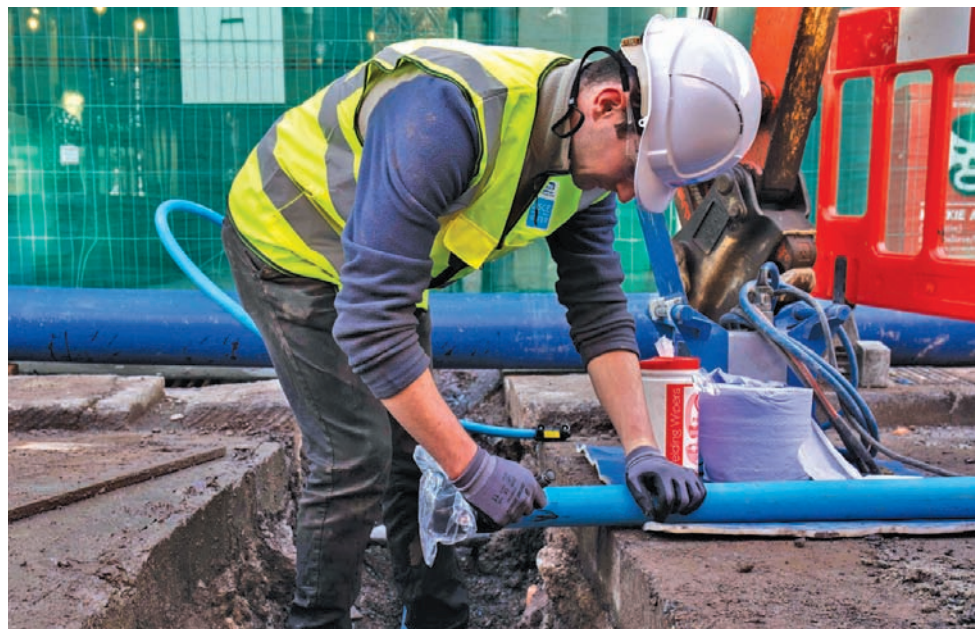
Irish Water, working in partnership with Wicklow County Council, is progressing with water main improvement works in Kindlestown, Greystones
