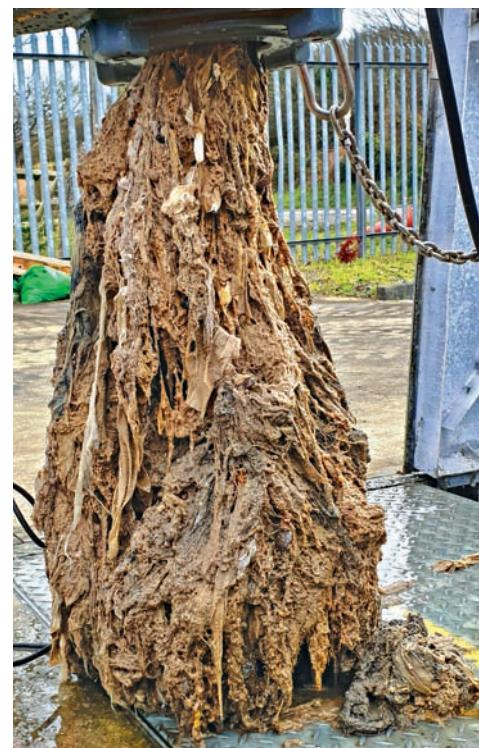
An 8ft blockage that was removed from the Bollarney Wastewater Pumping Station last year. The blockage serves as a reminder of the problems caused by inappropriate items being flushed down the toilet.
